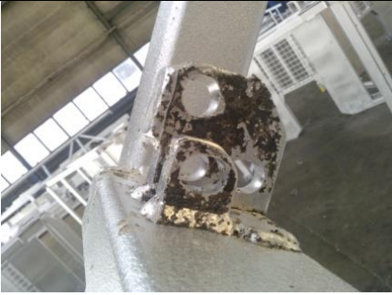
Impurities on steel, sticker marks resulting in lack of zinc plating – remain unpainted
